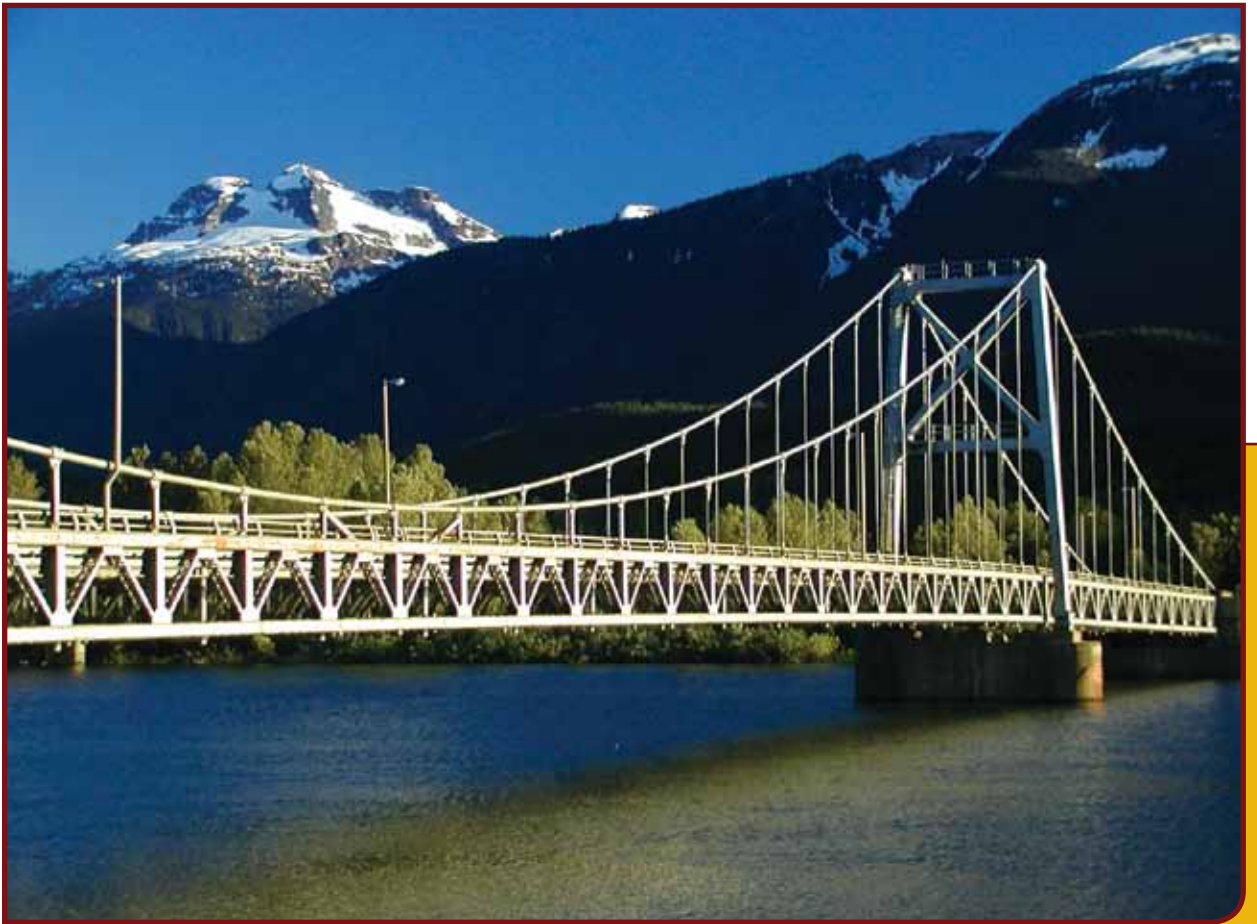
The Revelstoke Bridge, Photo: Courtesy of Evan Batke
