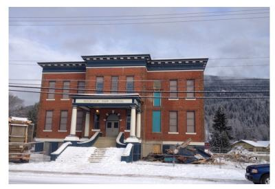
There was less damage to the front facade than anticipated. The photo shows the exterior staircase addition to the right of the front stairway removed, leaving the surrounding brick facade largely intact.
