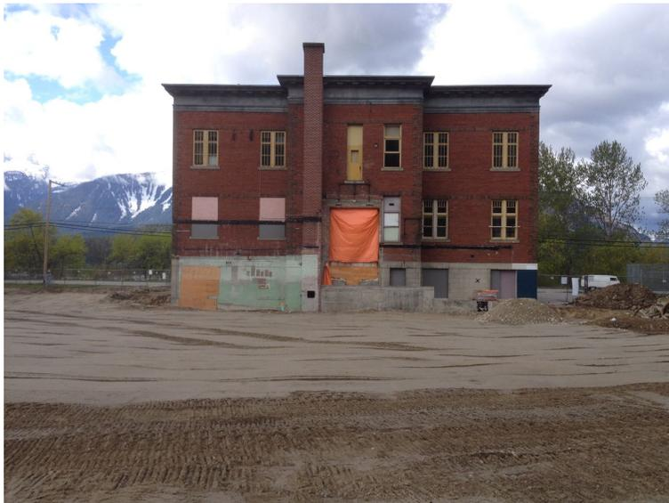
A small portion of foundation will remain to ensure the chimney is properly supported. Once repurposing of the building is confirmed, a decision can be made regarding the demolition of the chimney.
